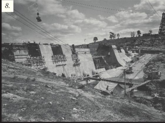
6. Gordon Dam in Tasmania is a double arch concrete dam. It escalates 140m and supports the States largest hydropower scheme, approved by Parliament in 1967. (TAS)
