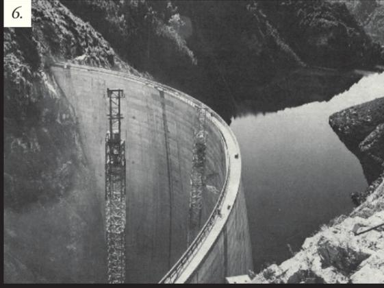
7. The Gordon Dam was constructed by from 1972-1974, consuming 154,000 cubic metres of concrete. In 2001, it was still the highest arch dam. (TAS)
