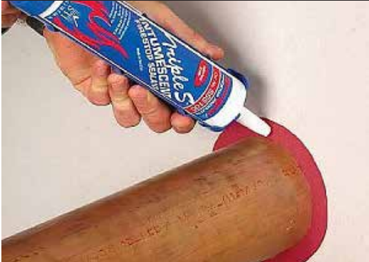
Typical fire caulk material sealing the openings around the systems.
