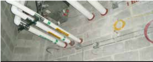
Typical fire caulk material sealing the openings around the systems.
