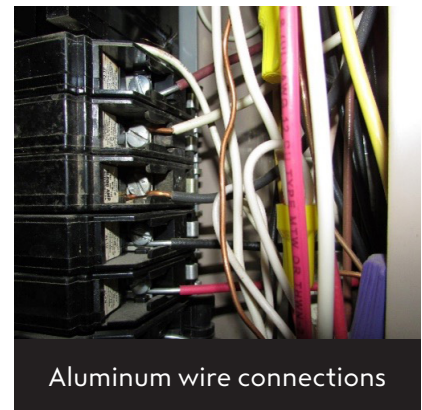
Aluminum neutral wires
